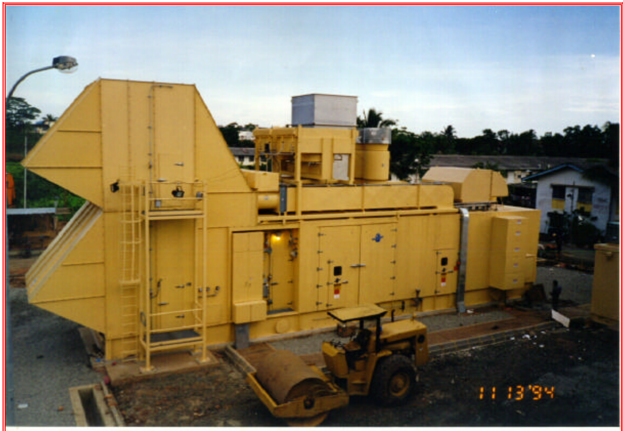
Figure 19 : LM2500 GTG simple cycle power plant that was engineered by Vy Consult
